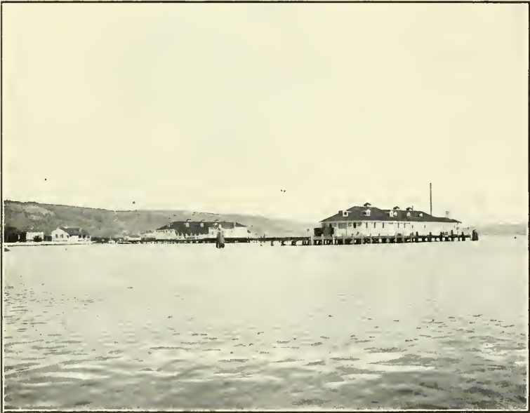
QUARANTINE STATION AND MARINE HOSPITAL AT LA PLAYA, SITE OF HIDE HOUSES
